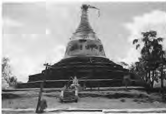
Figure 3: The umbrella of Maung-ti pagoda was broken, and ancient plasters on the bell-shaped dome were torn off. Maung-ti pagoda was built in lower Myanmar by King Anawrahtar of the Bagan kingdom in the 11 th century AD. It was of a peculiar architecture featuring a Bagan-type pagoda built on five receding terraces made of laterite stone blocks. (photo by Nyunt Han).
