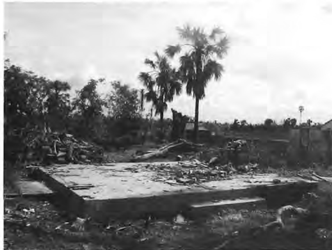
Figure 11: The scene of a wooden shrine totally blown away from the brick platform near Maung-ti pagoda in Twantay (photo by Nyunt Han).
