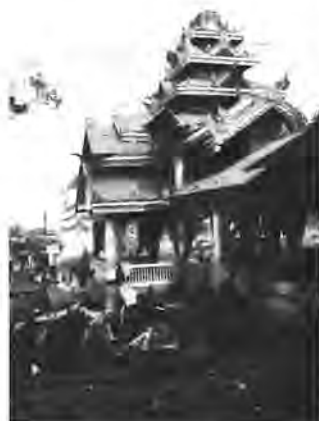
Figure 9(b): The view of a damaged entrance pavilion at Kyaik-khauk pagoda (photo courtesy of the Pagoda Trustee Committee).
