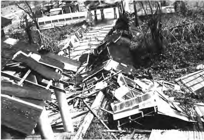
Figure 13: At Kyaik-khauk pagoda in Than-hlyin, the roof-covered stairway on the northern side collapsed to the ground. Many roofs of corrugated sheets were ripped off (photo courtesy of the Pagoda Trustee Committee).
