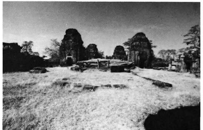
The remaining four of the five brick prang (towers). The middle, which is also the main prang, has already disintegrated.
