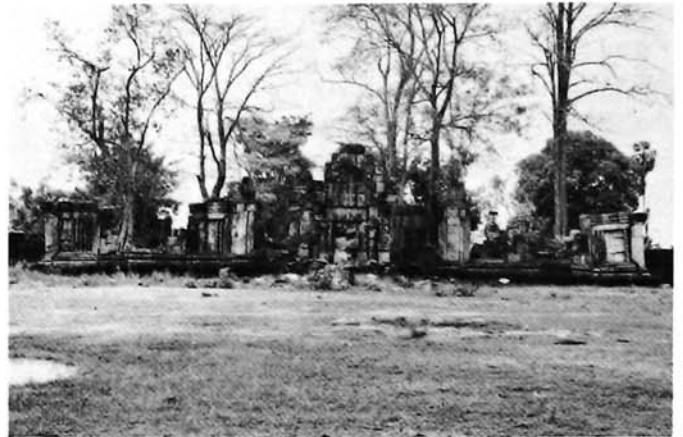
The southern gate of the outer wall is in style B. Its only entrance is flanked on both sides by a window with four balusters.
