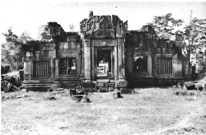
Eastern gate of the inner gallery flanked on each side by two balustraded windows.
