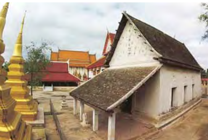
Exterior of temple (Wat Pa Klang Thung) prior to conservation efforts
