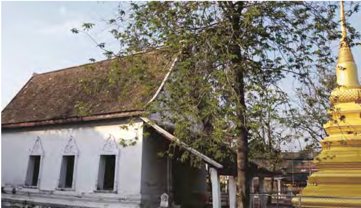
Temple exterior as work nears its end
