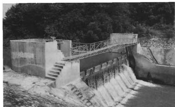
Upgraded French dam raises the water level in the canal to allow the water to enter through the old intake and fill the West Baray, which has been converted to a modern irrigation reservoir.
