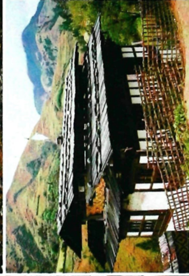
Traditional Bhutanese house with easily-replaceable wooden slat roof
