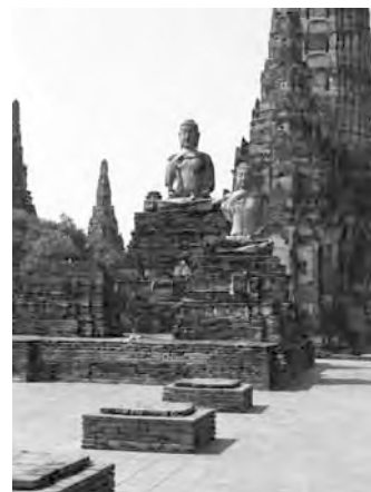
Ayutthaya, Wat Chaiwatanaram (2009)
