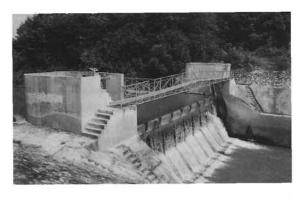
Upgraded French dam raises the water level in the canal to allow the water to enter through the old intake and fill the West Baray, which has been converted to a modern irrigation reservoir.
