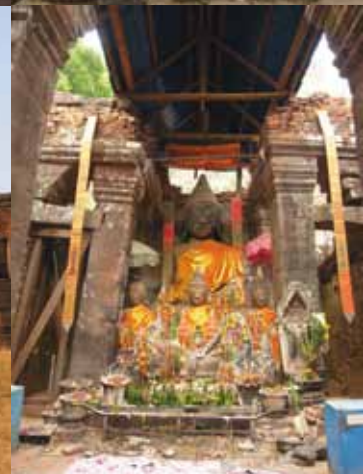
Vat Phou, Buddha statues inside the sanctuary covered by a recent roof (2008)
