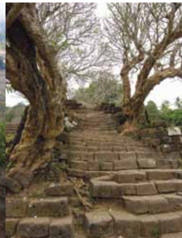
Vat Phou, stone stairs damaged by the tree roots (2009)
