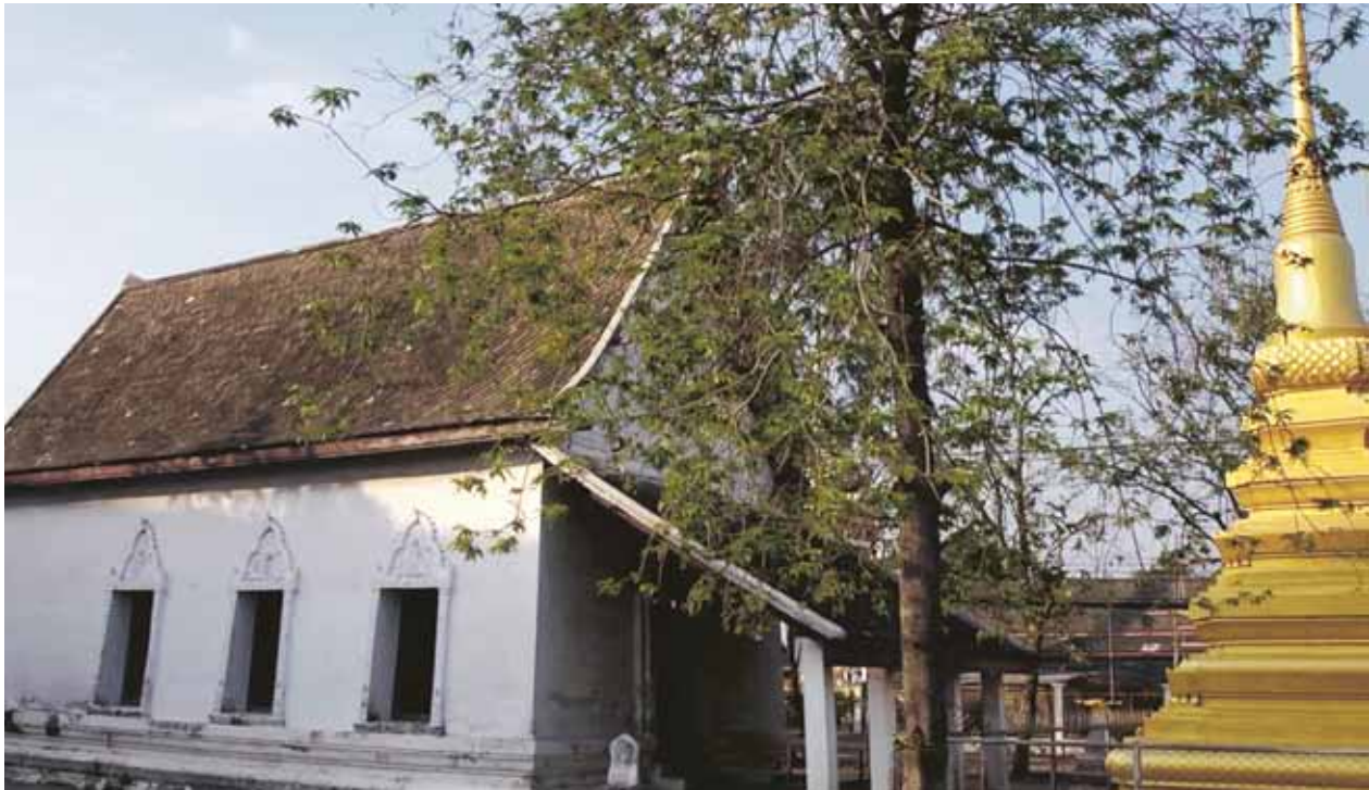
Temple exterior as work nears its end
