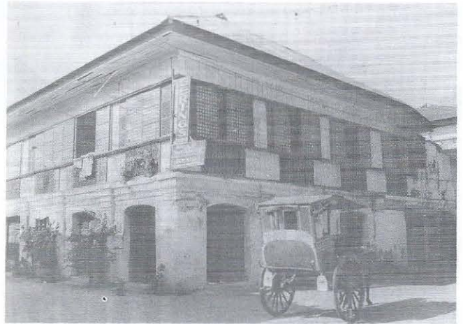
Thick walls, hardwood floors, high ceiling, tile roofs make these old houses of Vigan venerable looking and formidable as forts.
