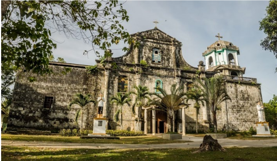
Fig. 13 Façade of Matalom Church. Source: Photograph by Dr. Bethlehem Ponce, 2019.
