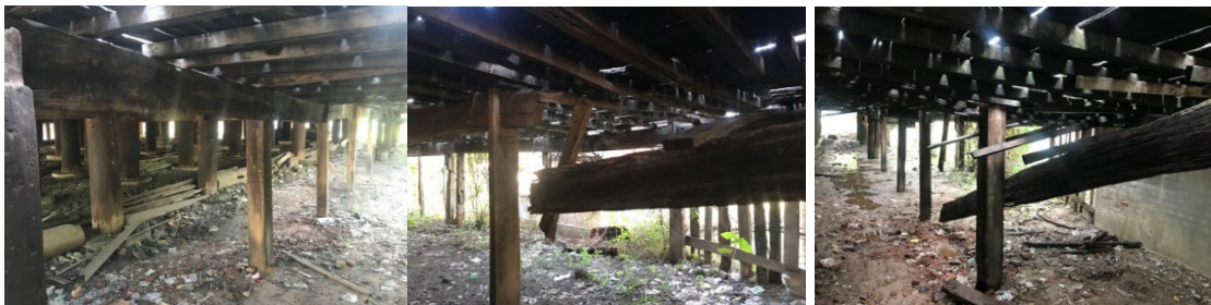
Fig. 11 Condition of main beam under the north veranda in January 2020, in October 2021 and in September 2022. Source: Photos by author.
