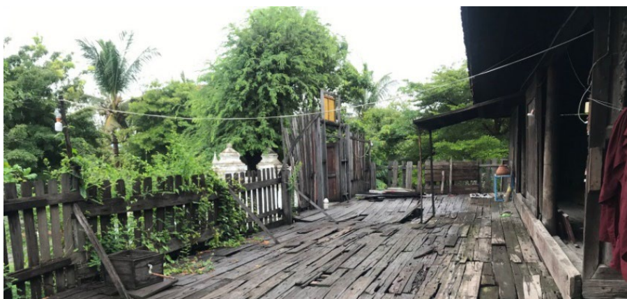
Fig. 10 Condition of veranda floor. Source: Photo by author, 2022.
