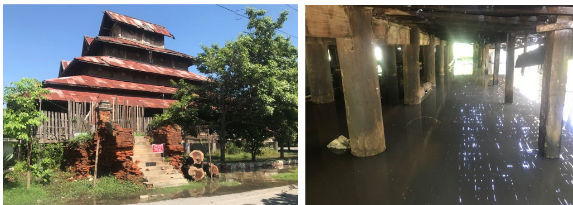
Fig. 6 Flooding around and under Maha-Minhtin monastery. Source: Photo by author, 2021.
