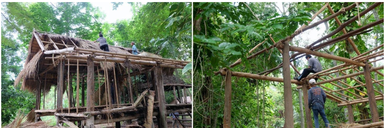
Fig. 10 There were several houses on site. One or two carpenters usually worked on one building. From time to time, the team member or senior carpenter would go check on the work. Source: Photo by Hiranpruek, 2017.
