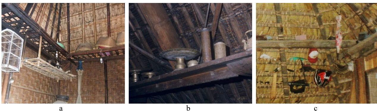
Fig. 8 Tie beams which doubles as storage shelf: a) in a Sasak house at Sade village, Lombok, b) in a Toba Batak house, c) in a Sawu ammu pe house documented by Athasya Kandhiya. Source: Midori (2010), Tropenmuseum and Lawson (1971), Mosmarth et al (2017: 56).
